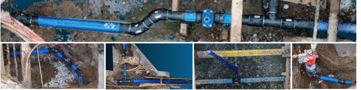
Fig. 3: 3D reconstructions of excavation sites from our data set, depicting the predominant use of straight pipes and T-junctions. When hard pipes are used for water or gas, they show only sharp angles of 45^\circ , 60^\circ , or 90^\circ , as shown in the bottom left image. Some reconstructions also show a small outgoing branch, as seen in the top image. Occasionally, pipes are partially covered by dirt, as shown in the bottom row, third image.
